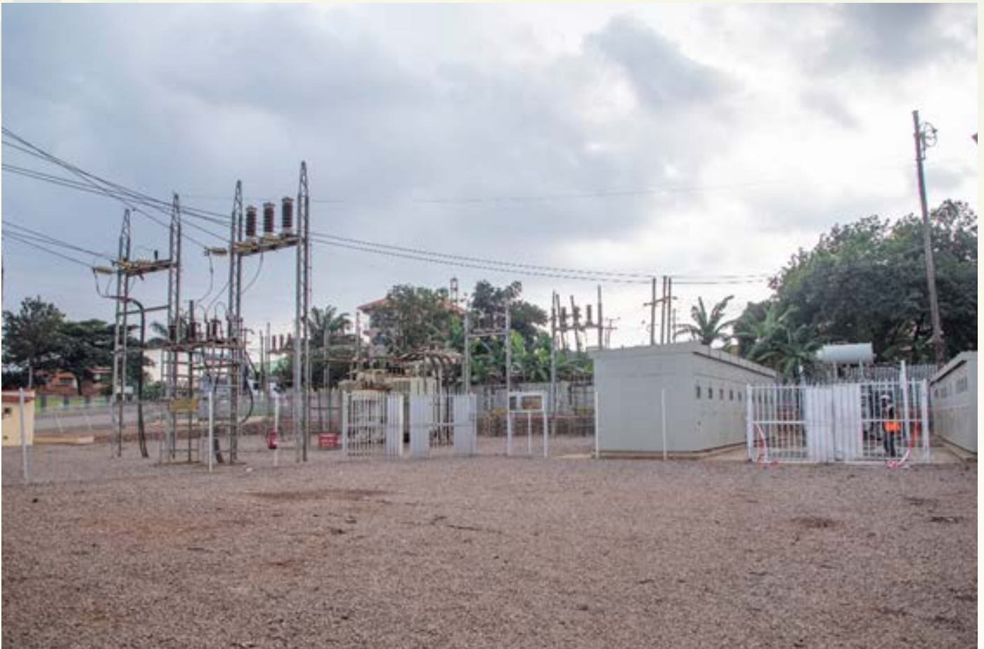
A wide view of the Kampala South Substation following its upgrade from 20MW to 34MW
