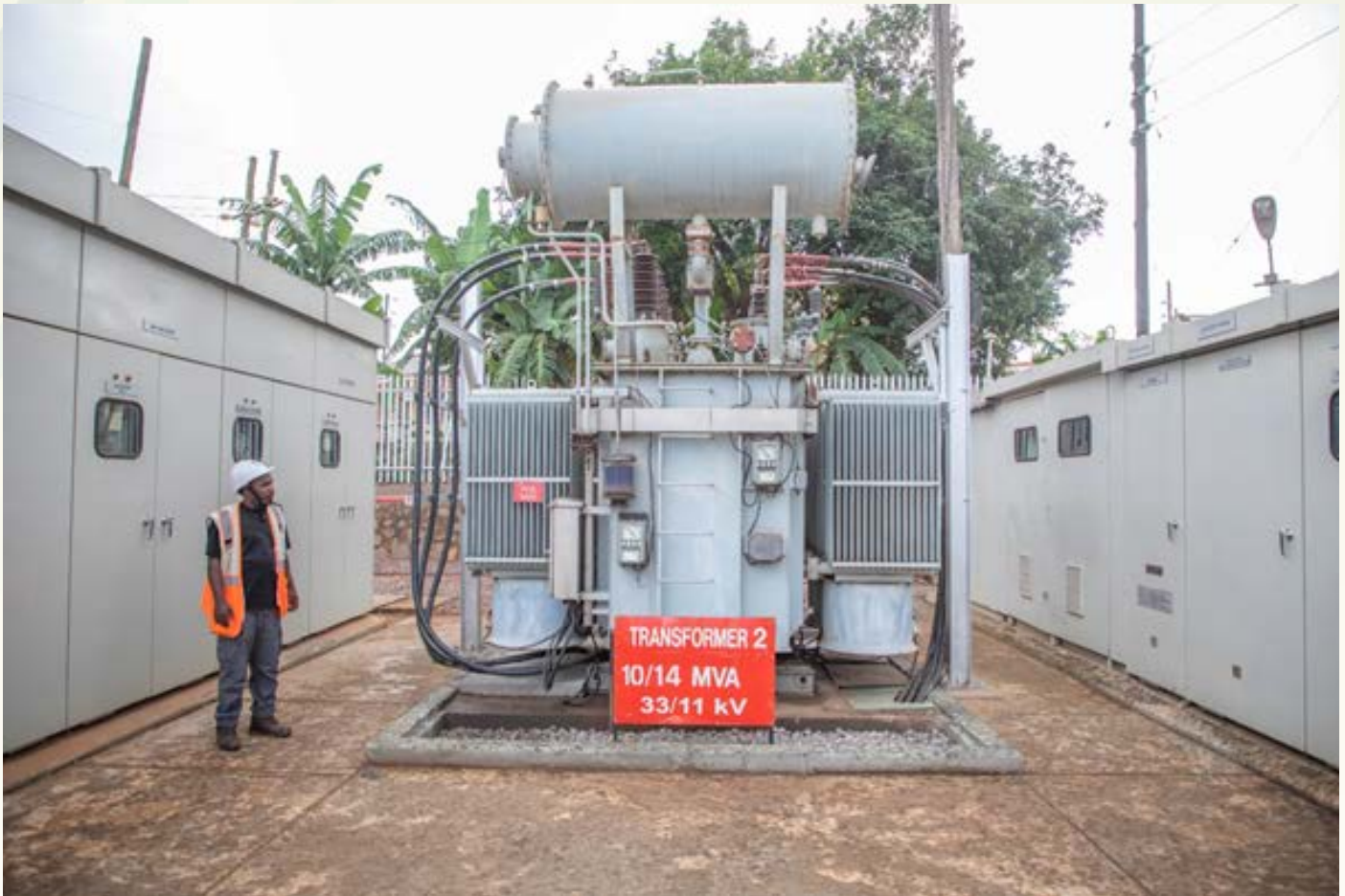
The newly installed 10/14 MVA, 33/11kV transformer at Kampala South Substation
